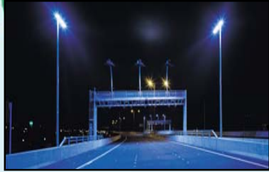
Australia - Melbourne City Link Project
